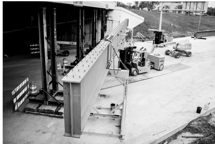
| 2013 SOUTH SPLIT PROJECT
