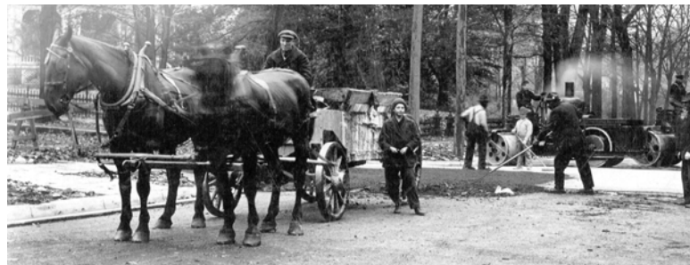
PHOTOS PROVIDED BY BROOKS CONSTRUCTION; 1917 ASPHALT PLANT AND ROAD WORK
