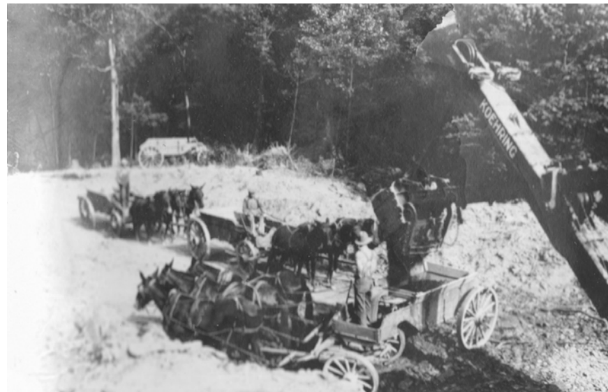
| 1928 HEAVY GRADING EAST OF SALEM ON STATE ROAD 56
