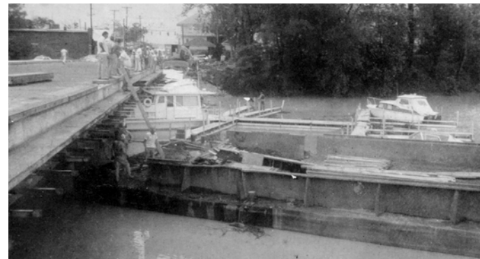
JUNE 10, 1981 BARGE STUCK UNDER HOGAN CREEK BRIDGE, STATE ROAD 350 AND LOOKING TOWARD US 50
