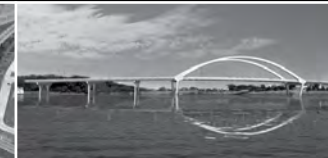
Hastings Bridge Design-Build — Hastings, Minnesota
