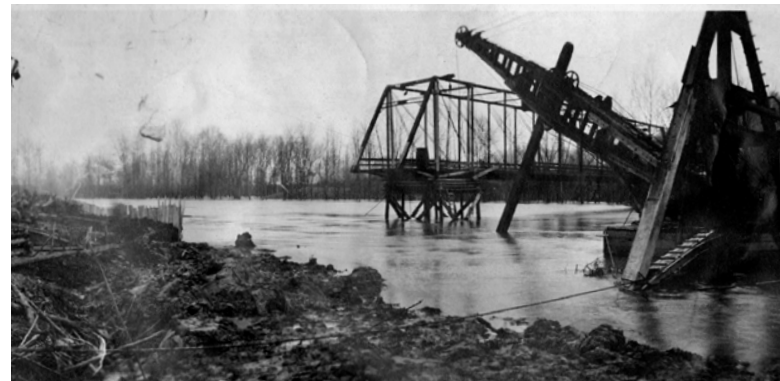
| DECEMBER 2, 1921 ORIGINAL MILTON-MADISON BRIDGE CONSTRUCTION
