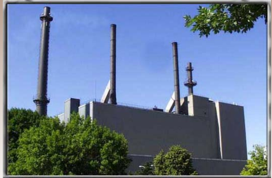
Wade Utility Plant, Purdue University
