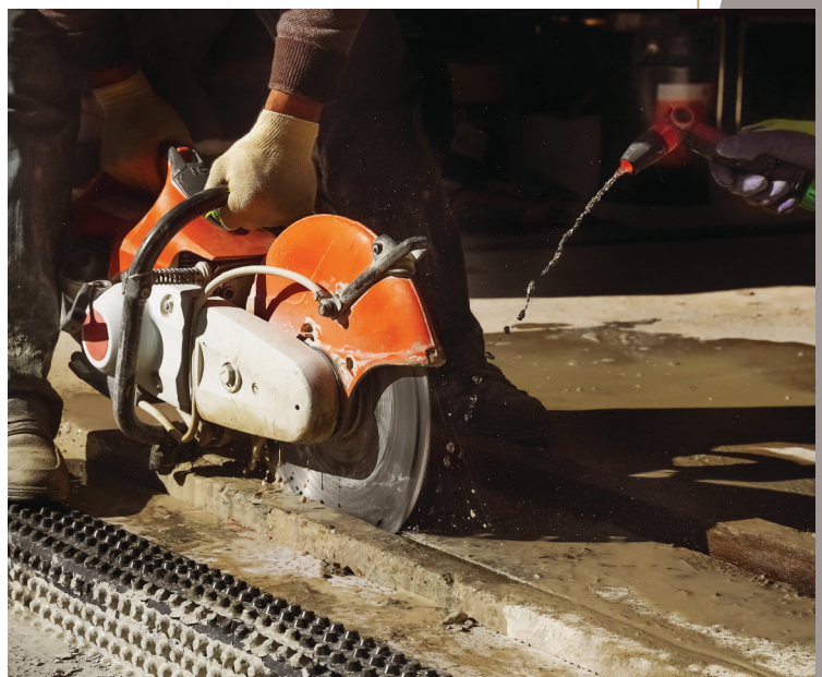
A worker wet-cutting concrete to reduce silica dust presence
