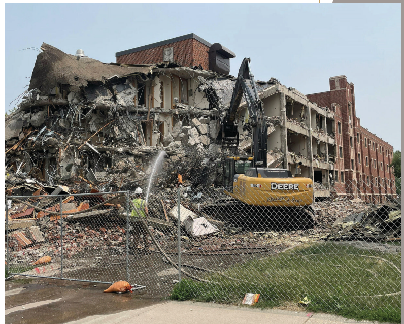
Demolition of a campus building
