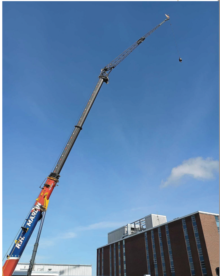
Example of a crane on site
