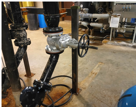
An example of a utility shutoff.
