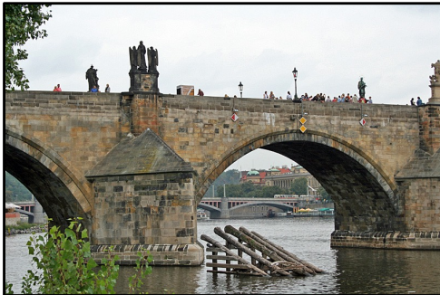
Charles Bridge, 1357 (arch structure)
