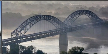
Sherman Minton Bridge (truss-cable structure)
