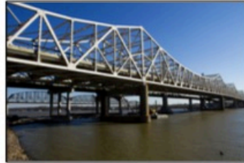
Kennedy Bridge (truss structure)
