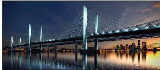
Lincoln Bridge (cable-stayed structure)
