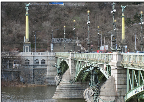
Cechuv Bridge, 1905 (truss substructure)
