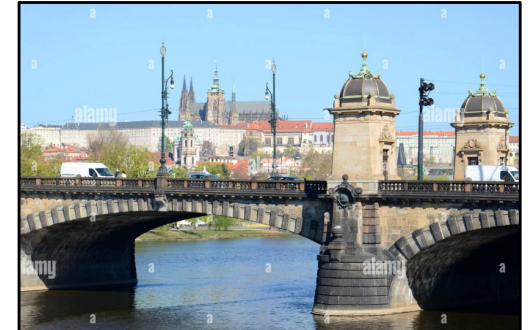
Legion Bridge, 1899 (arch structure)
