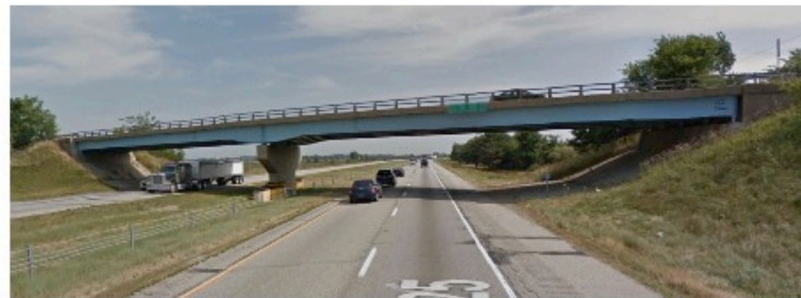
highway overpass bridge
