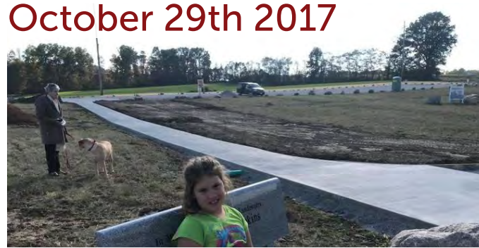
Accessible path was poured to access Picnic Shelter
